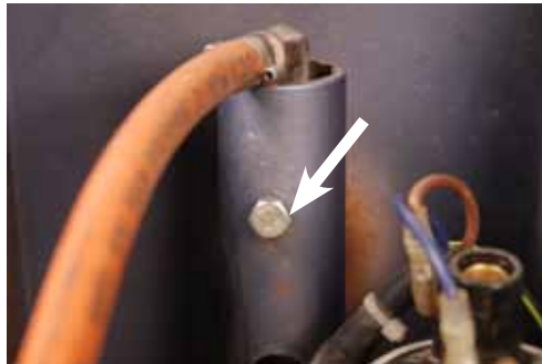
Figure 5. Hexagonal bolt retaining the gas injector in the firing tube.
